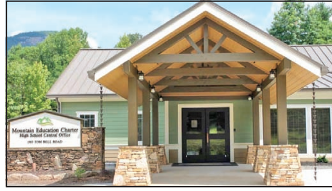
The new Central Office building for the Mountain Education Charter High School in Cleveland.
